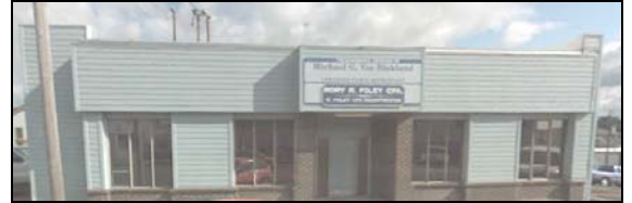
Van Blokland and Foley Building
